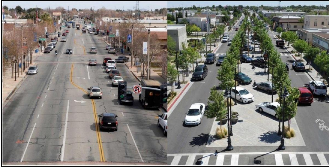
Figure 5: Before and after installation of a median chicane in Lancaster, CA.
